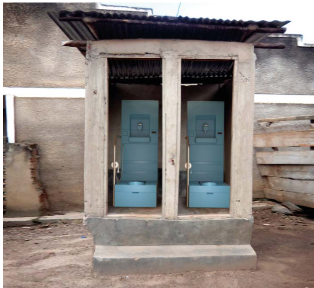
Figure 1: Photomontage @ EOOS- The Blue Diversion Toilet retrofitted into an existing pit latrine
